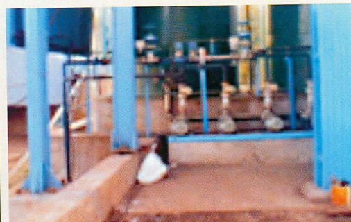
Hexavalent chromium removal treatment setup at the chrome ore beneficiation plant, in Sukinda (Odisha)
