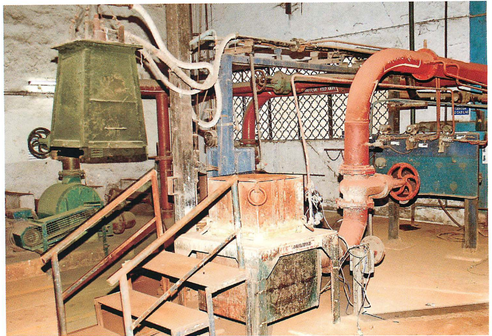
Pilot scale sintering facility at Tata Steel R&D
