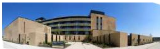
South side of the new building at West Cambridge, October 2013
